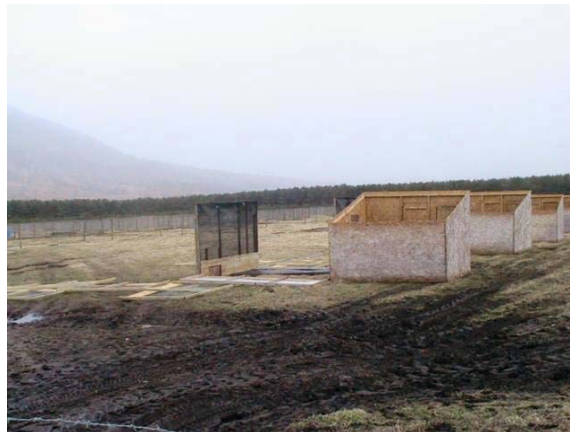
Fig. 6 : Game pens in construction (3/4/06)
